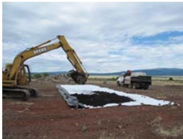
Figure 7. Construction of IXP<sup>ER</sup> 70C enhanced aerobic bioremediation soil treatment pile on liner (July 2012)
