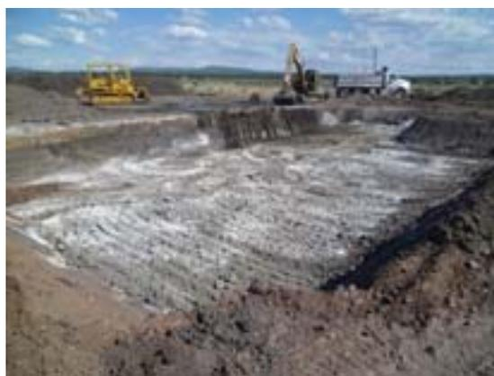
Figure 5. IXP<sup>ER</sup>® 70C Calcium Peroxide placed in the bottom of the completed former shop area excavation (July 2012)
