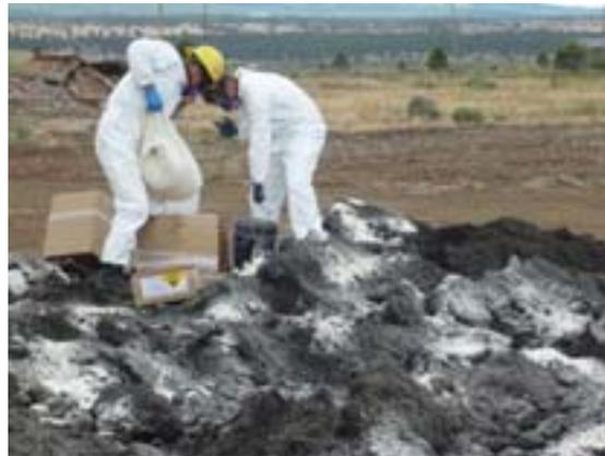
Figure 6. IXP<sup>ER</sup> 70C Calcium Peroxide being added to the soil treatment pile (July 2012)
